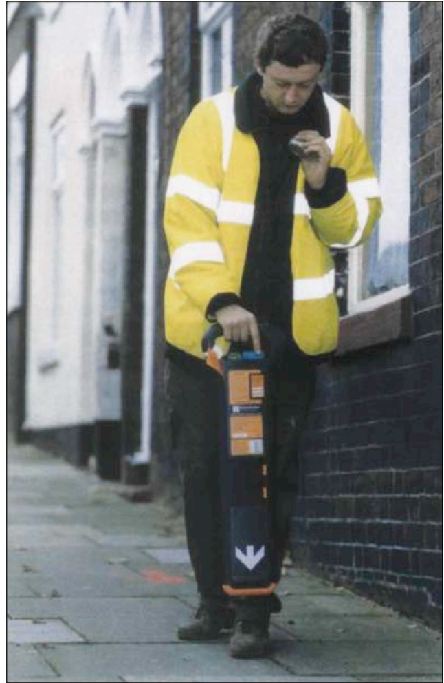
Figure 5 Using a cable locator
