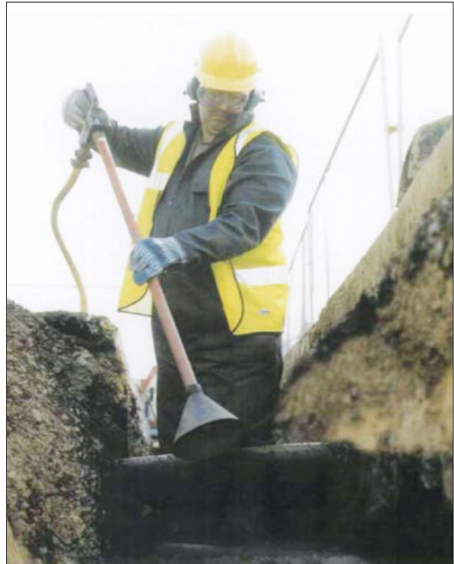
Figure 7 Using an air digging tool
