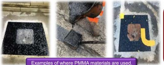
PMMA's must be finished with a suitable treatment to provide the necessary skid resistance. This may be bitumen coated chips or calcined bauxite to the specified PSV. You can see from the images where pre-coated chippings have been applied.
