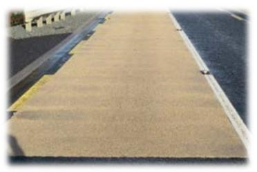
Reinstatement edges should be sawcut to 40mm depth. A bond coat must be applied in all instances. Edge sealant must be applied to top 100mm.
