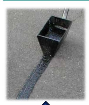
Overbanding being applied as a hot material poured into a shoe to provide the correct width un road surface.
