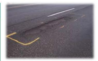
If undercutting occurs, and bound materials are not cut back as shown in Figure S6.5 it is likely to cause existing surface to fail at a later stage, as seen in the above image.
