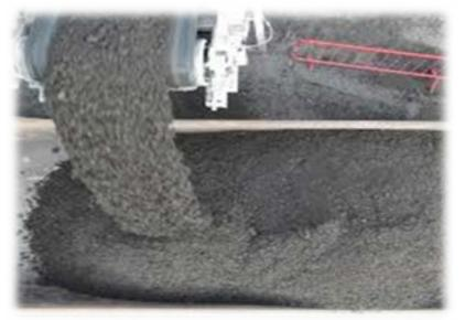
Image shows CBGM material being fed into trench ready for compaction.
