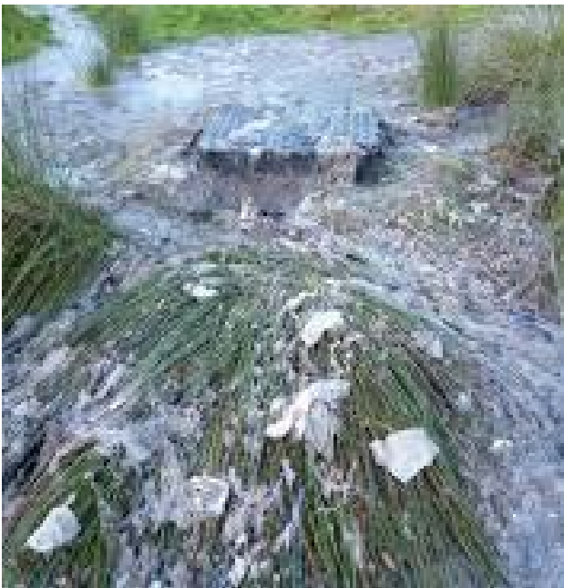
Above: Discharge of Water on to Public Highways
