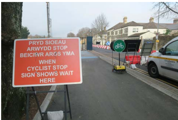
Above and right: Cycle lane maintained through roadworks
