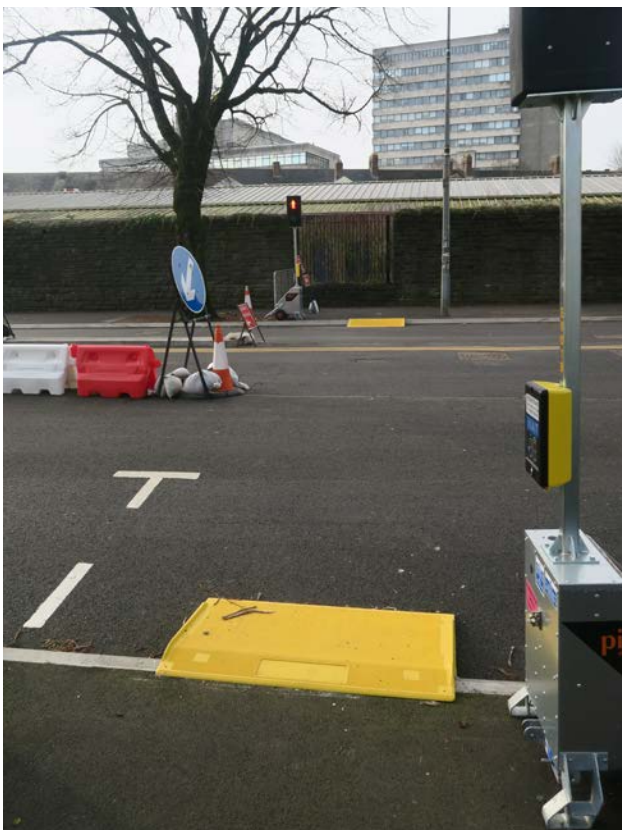
Above and right: Temporary footway ramps used on walking routes
