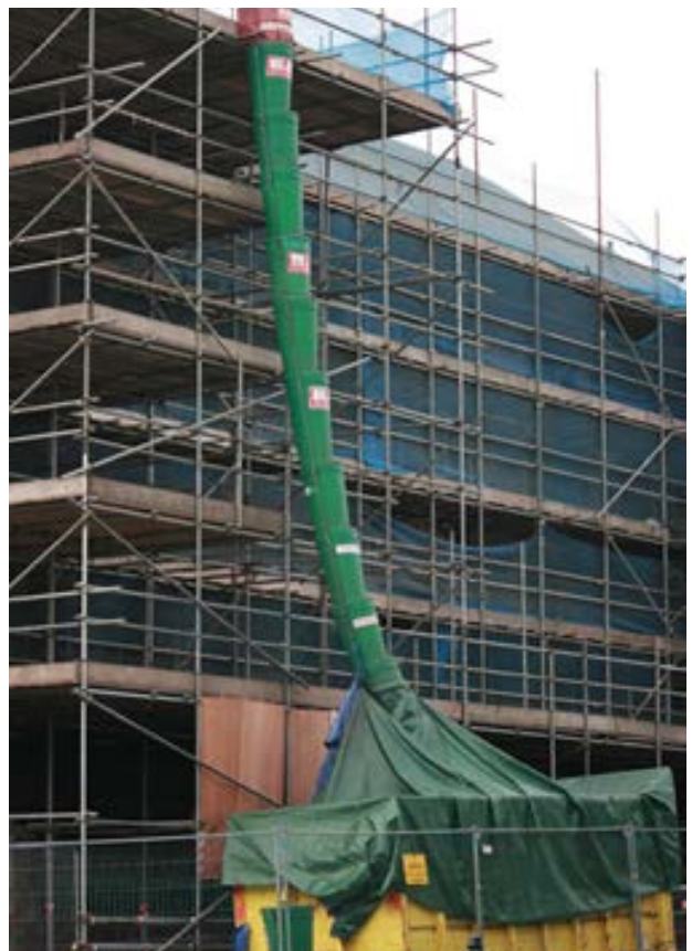
Above: Skips and Scaffolding
